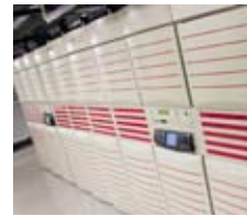
Clearfield Transmitter Site
