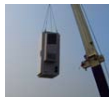
Base Station Installation
