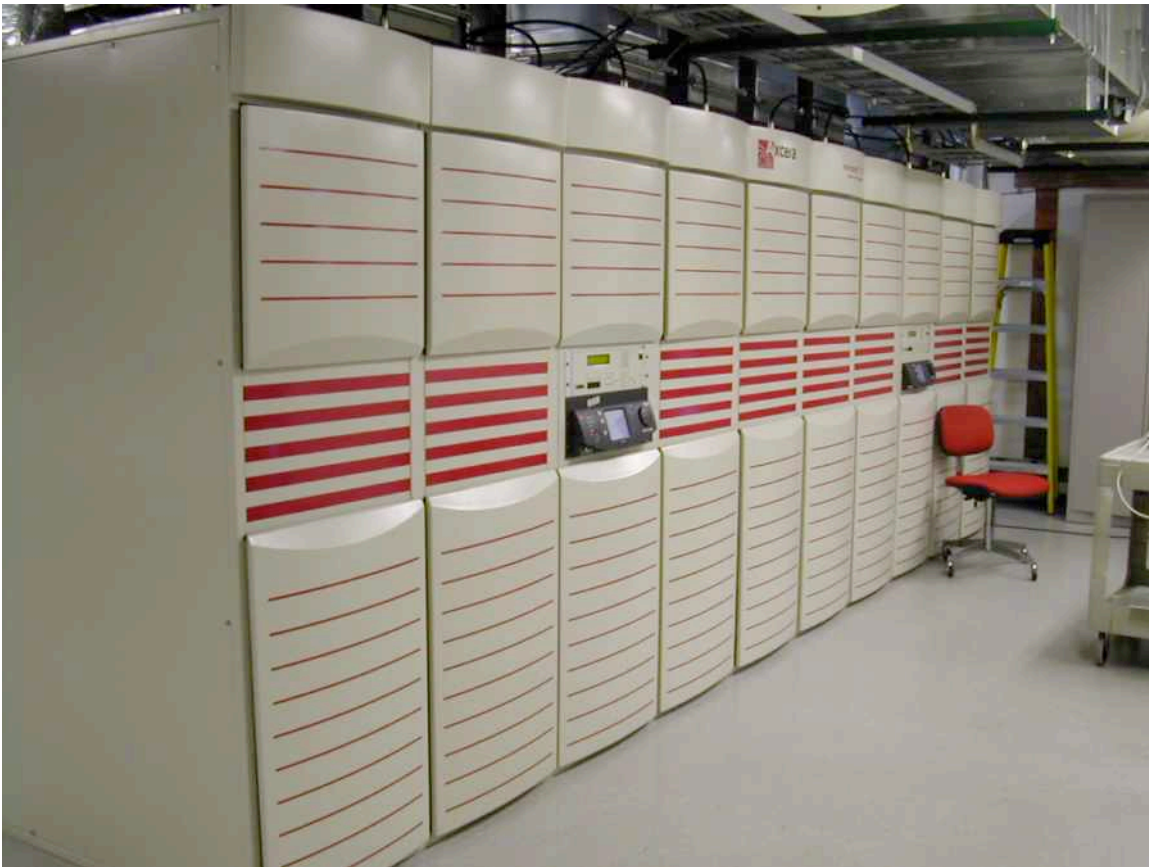
Figure 16 – Main WPSX (Distributed) Transmitter
